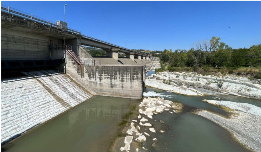
Figure 8. Hydraulic node of the Castellarano Weir
